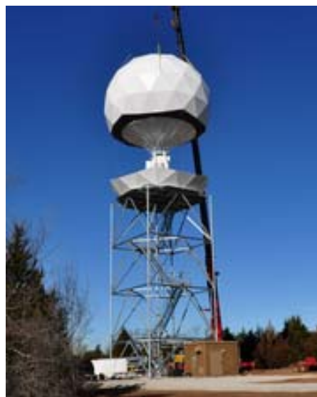
Figure 2-1 A weather radar for rainfall detection. ( http://en.wikipedia.org/wiki/Weather_radar )
