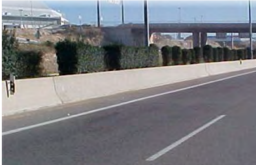
Figura 68. Barrera New Jersey “In situ”
