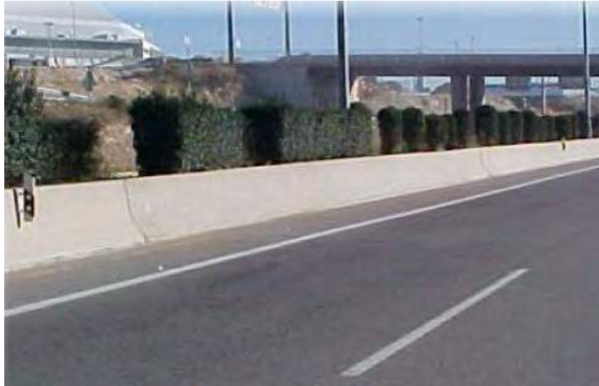
Figura 68. Barrera New Jersey “In situ”
