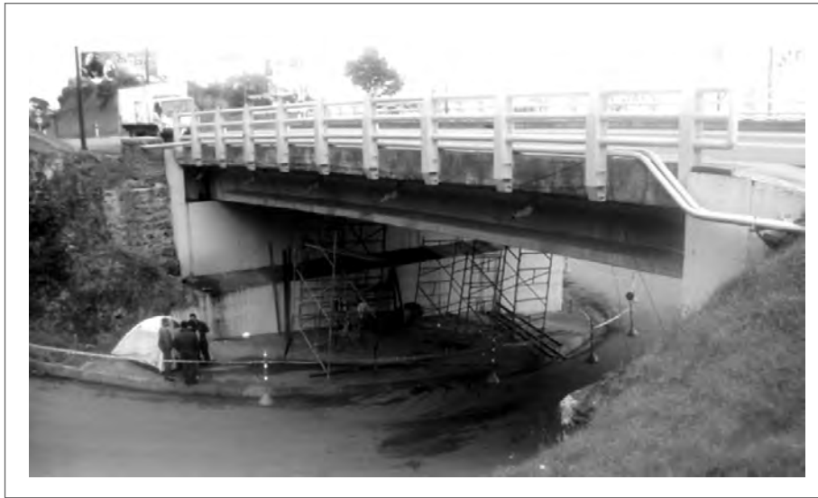
Figura 3. Vista en perfil del puente Boquerón simplemente apoyado de viga postensada y losa en concreto reforzado Figure 3. Cross section view for Boquerón Bridge, which is simply supported by a post-tensioned beam and reinforced concrete slab
