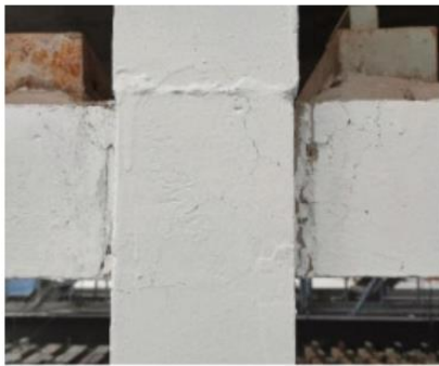
(a) Side beam-column joint
