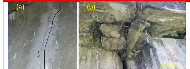
Figure 10. Visual condition of a deteriorated bridge. (a) side-view of post-tensioned beam; (b) local damage at beam joint. Source: Own elaboration
