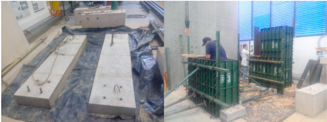
Fig. 2. Left: foundation and right: formwork.
