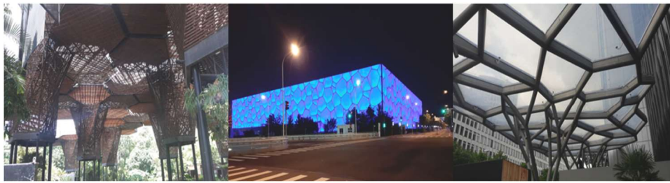
Fig. 3. Examples of structures with Voronoi configurations.
