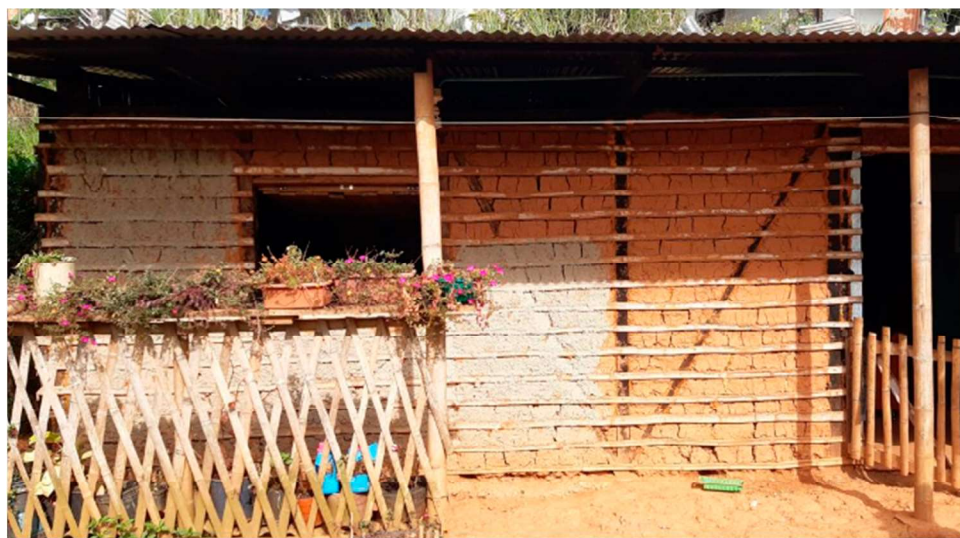
Figure 1. Example of bahareque wall in a typical house of the Estrella Community in the Jamundí District (Valle del Cauca, Colombia).
