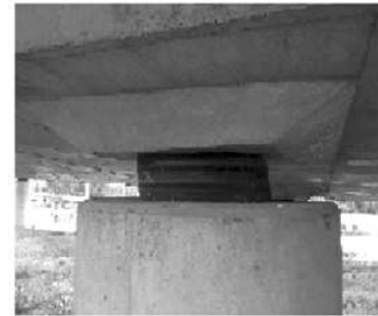
Figure 4. Connection of the bridge in the support and the bearings. Source: [13]
