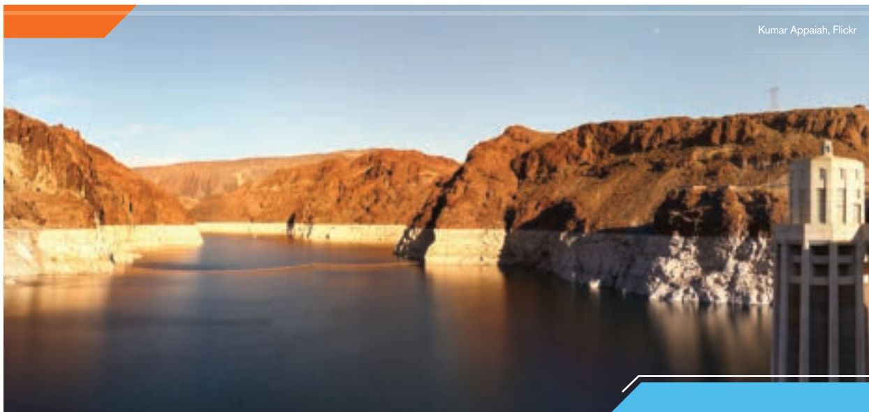
Lake Mead near Hoover Dam, Nevada, USA
