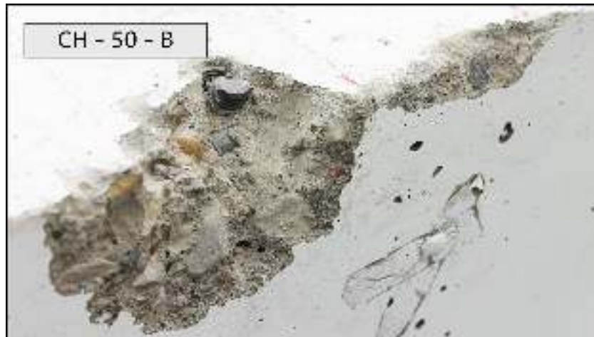
Figure 84 Failure mechanism CH – 50 – B*. Source: Own.
