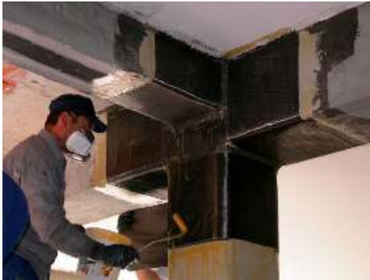
Figure 3 Strengthening of a beam-column connection with FRP laminates. Source: (Rendón, 2016, p. 121)
