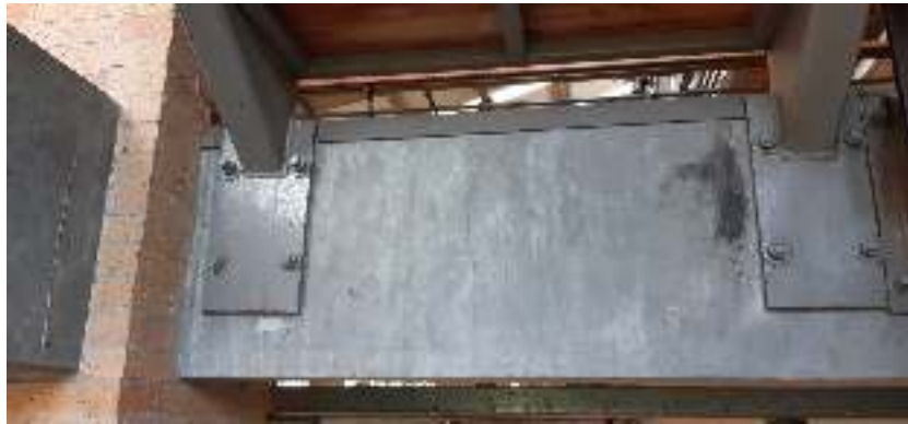
Figure 4 Steel staircase connected and supported by a concrete beam. Source: Own.
