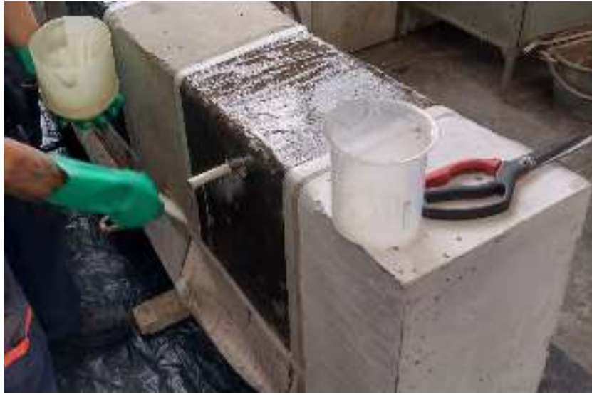
Figure 32 Application of filling putty to guarantee uniformity of the concrete region in contact with the CFRP. Source: Own.
