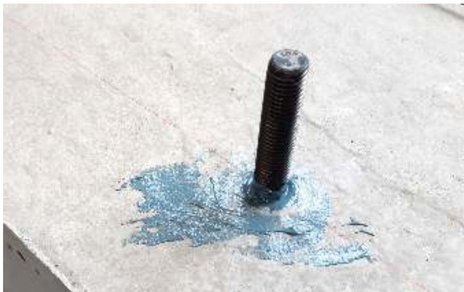
Figure 18 Installation of a bonded anchor. Source: Own.
