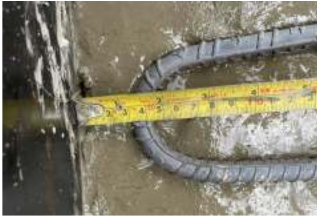
Figure 30 Hairpin installation to guarantee contact with the anchor. Source: Own.
