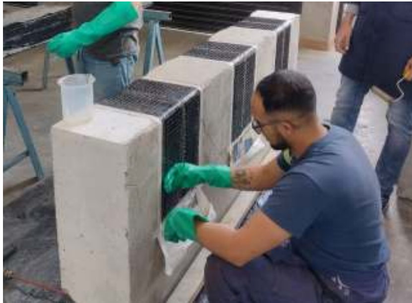
Figure 33 CFRP installation. Source: Own.
