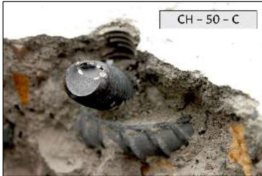
Figure 85 Failure mode CH – 50 – C*. Source: Own.
