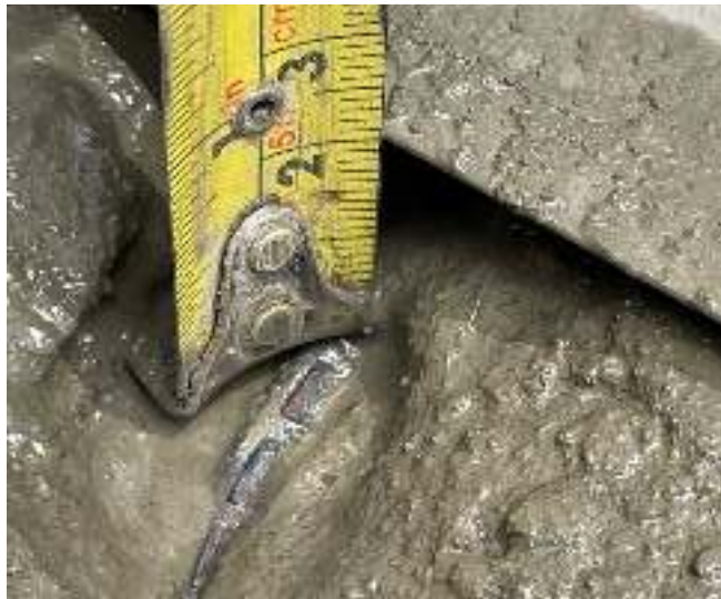
Figure 31 Hairpin installation guaranteeing minimum concrete cover. Source: Own.
