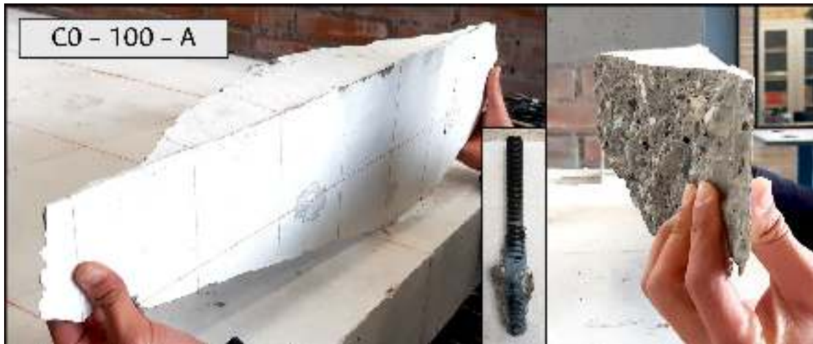
Figure 26 Concrete breakout body C0 – 100 – A. Source: Own.
