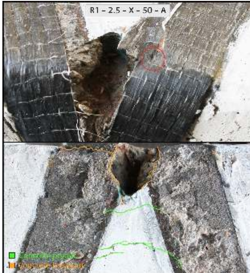
Figure 98 Failure mode R1 – 2.5 – X – 50 – A*. Source: Own.
