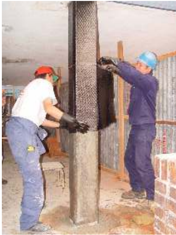
Figure 2 FRP jacketing of a column. Source: (Rendón, 2016, p. 18)
