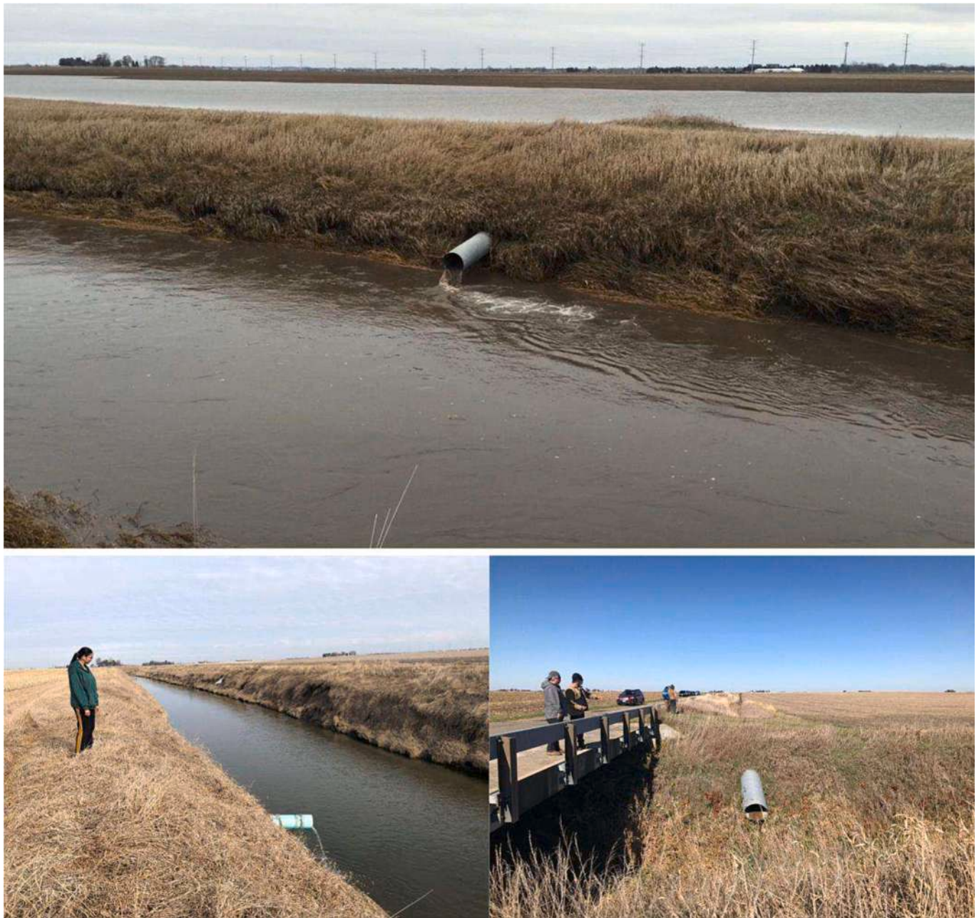
Fig. 3. (top) runoff from a low-gradient farmed hillslope impounded behind an artificial levee along a drainage ditch with ponded water draining into the ditch through a surface drain, (bottom left) subsurface tile draining into a drainage ditch with steep eroding banks, (bottom right) roadside ditch connected to a drainage ditch via a pipe through ditch levee at a bridge crossing.
