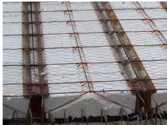
Fig. 1. Slab panel before cast-in-place concrete.
