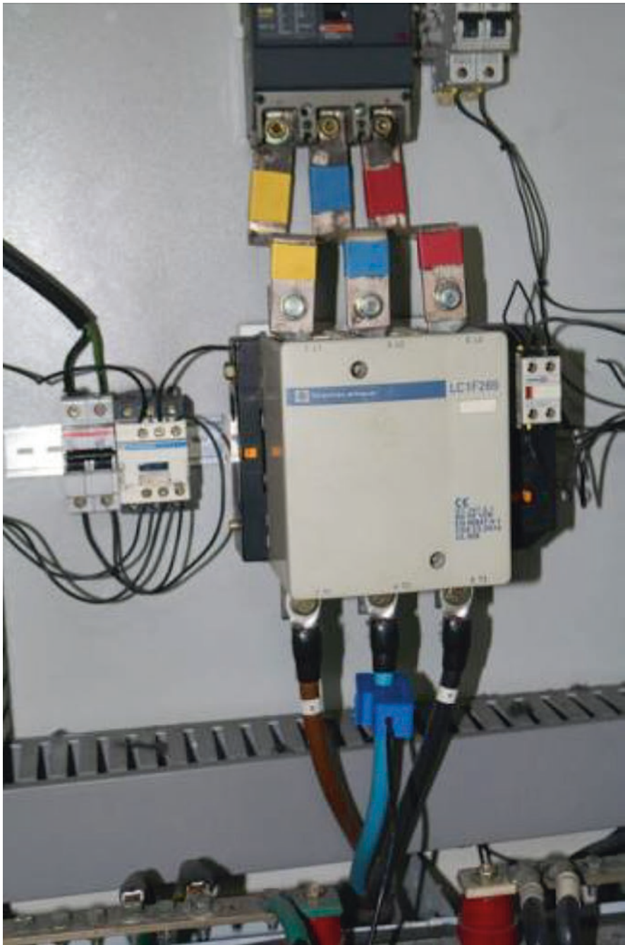
Fig. 7 Installing the current sensor
