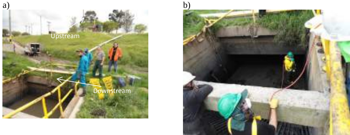
Figure 3.15 Hydraulic system. a) Upstream and downstream section of the discharge tunnel; b) entry to the discharge tunnel
